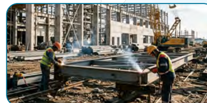
Vietnam Under construction in 2026
