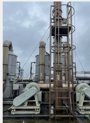
Acid/ Alkali Exhaust Gas Scrubber Equipment in Taiwan Plants
