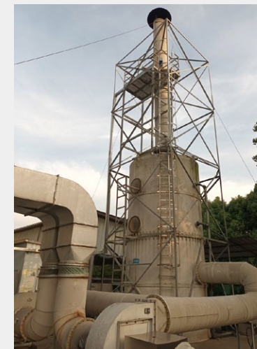
Spray Absorption Tower Equipment in Wuxi Plant
