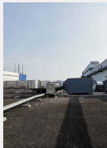
Organic Exhaust Gas Equipment in Chengdu Plant
